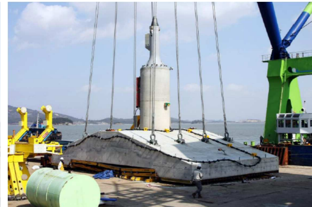
Gravity base foundation prototype [RENETEC & Ed. Züblin AG]
