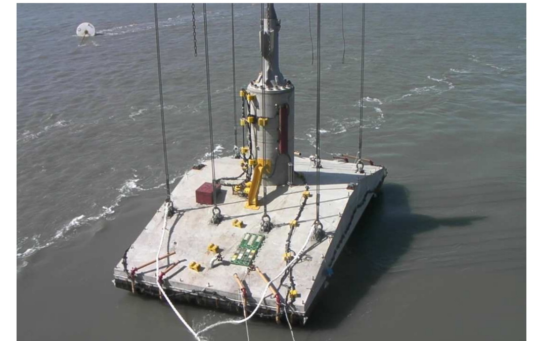
Foundation installation at the project site [RENETEC & Ed. Züblin AG]
