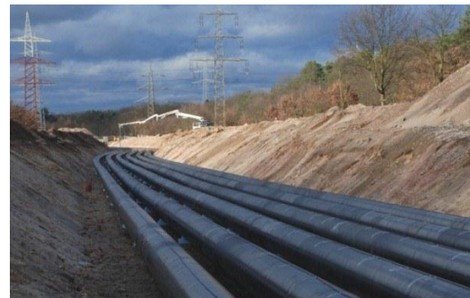
Figure 1: Trench with GIL phases
