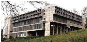
Fig.113 View of the La Tourette
