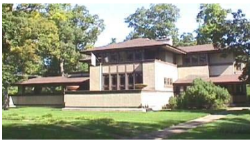
Fig.108 View of the Willits House
