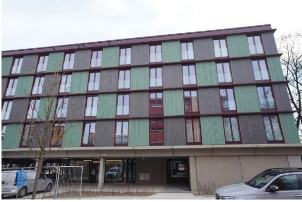
Fig. 3: Sample from the FaMatMuc dataset: The image has a resolution of 5304 x 7952 pixels and shows the front view perspective of a five-story residential building with a concrete base and a timber main facade
