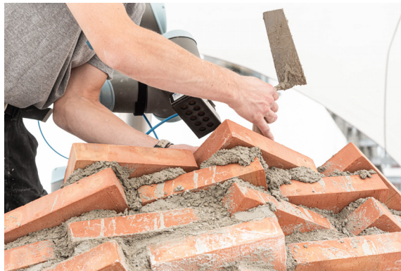
(b) Bricklayer knocks the brick into the mortar
