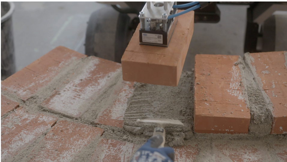
(b) The mason applies the mortar before the robot places the brick
