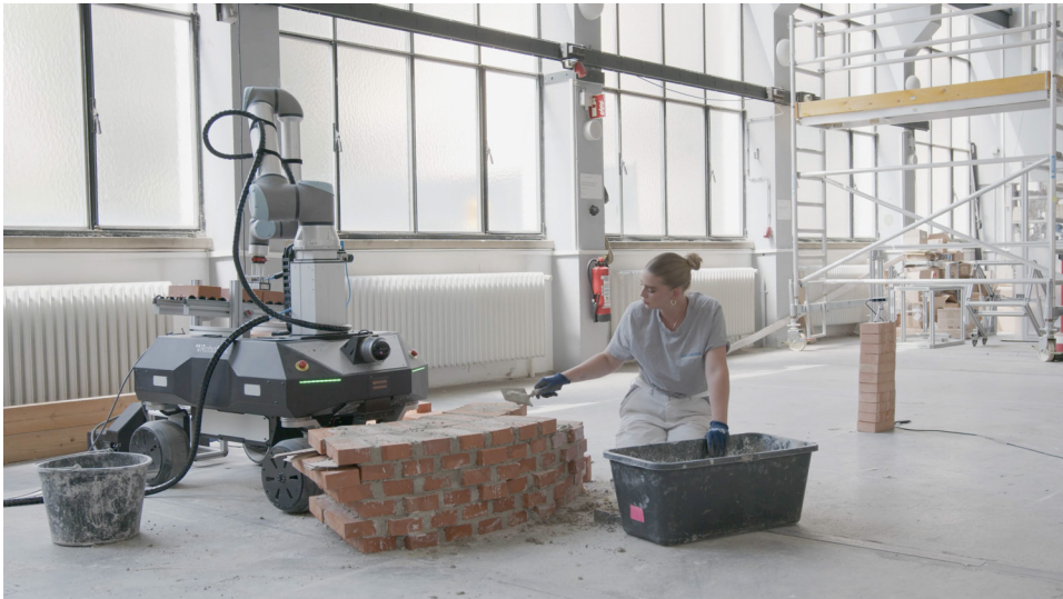
(b) The mason applies the mortar, taps the bricks into place, and cleans the joints
