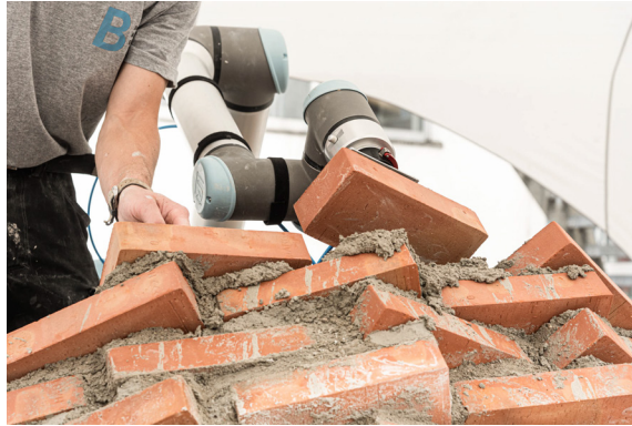
(a) The robot places a brick
