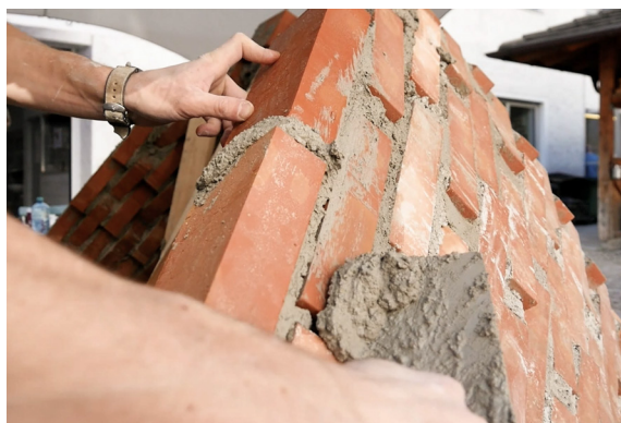
(c) Bricklayer cleans the mortar
