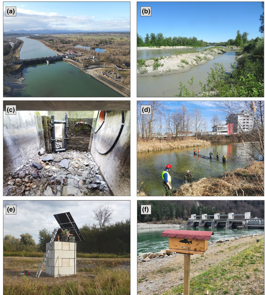
FIGURE 2 Photographs of (a) the River Inn at the Feldkirchen hydropower plant, (b) bank habitat restoration at the Rosenheim hydropower plant, (c) installed antenna in pass-through-orientation in the fish pass Teufelsbruck, (d) antenna installation in pass-over-orientation in the Mangfall tributary, (e) stationary detection station with solar system to power one of the antennas in the Perach fish pass, (f) mobile scanning stations for recreational anglers at the Teufelsbruck hydropower plant.
