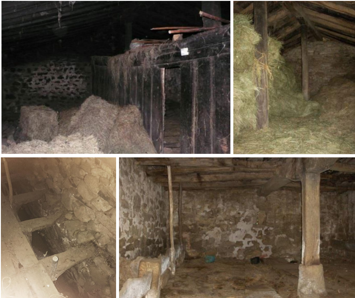
Figure 14: Impressions of the interior space, clockwise from the top left: upper floor with partitions, upper floor, gap used to throw hay down to the feeders, ground floor
