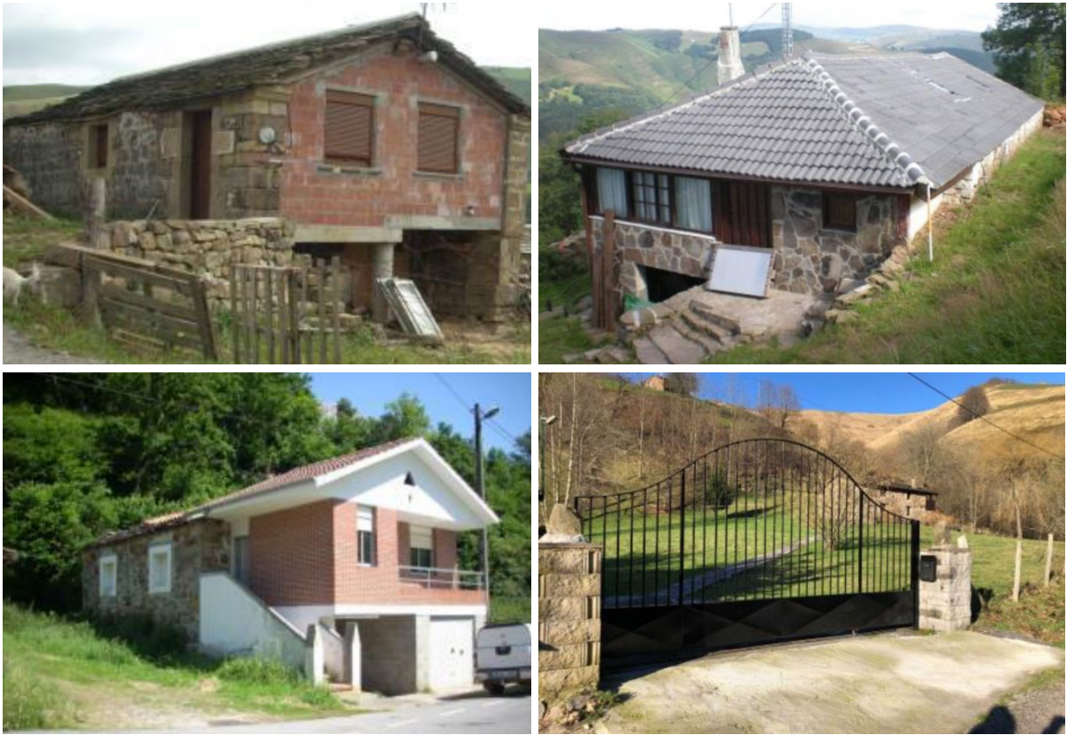
Figure 3: Examples of renovations that profoundly alter the traditional character of the cabaña pasiega
