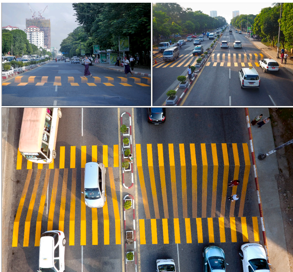
Fig. 2. The 3D crosswalk painted in urban Yangon (top left: drivers' perspective; top right: bird's eye view; bottom: top view).
