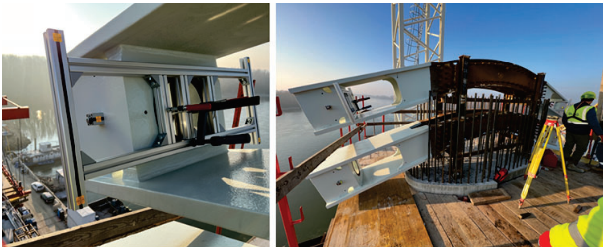
Figure 12: Setting passive anchoring link elements on top of the pylon
