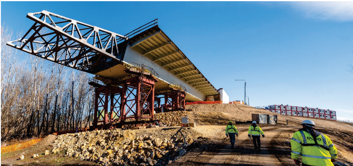
Figure 5: Left floodplain bridge during longitudinal launching (foto: Tamas Dernovics, magyarepitok.hu)
