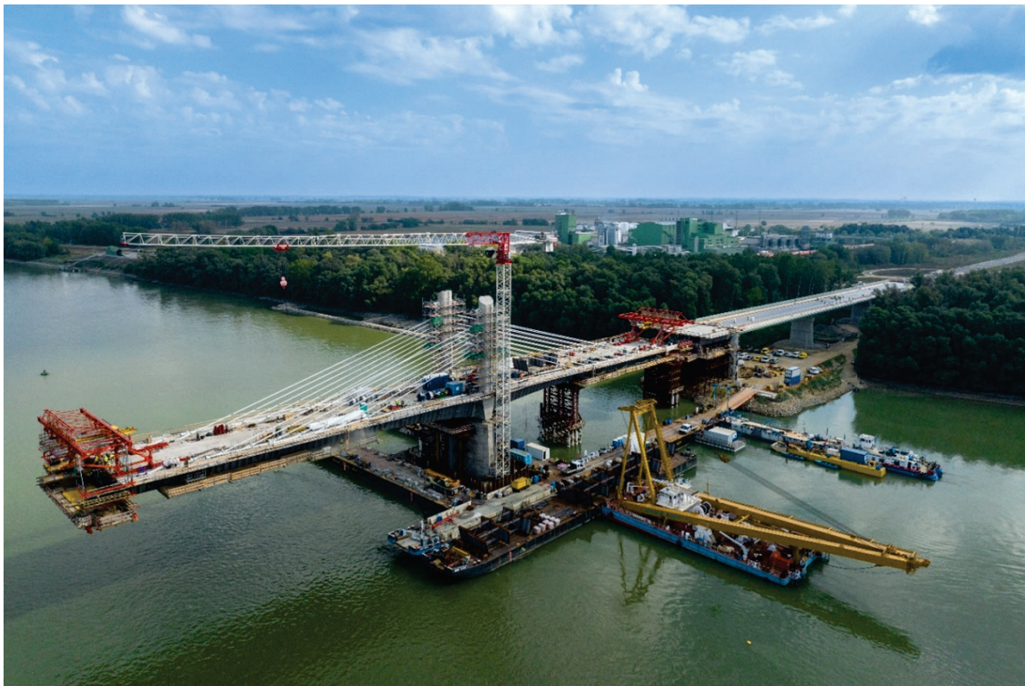
Figure 8: Cantilever construction of the river bridge (photo: Mihaly Erdei, magyarepitok.hu)
