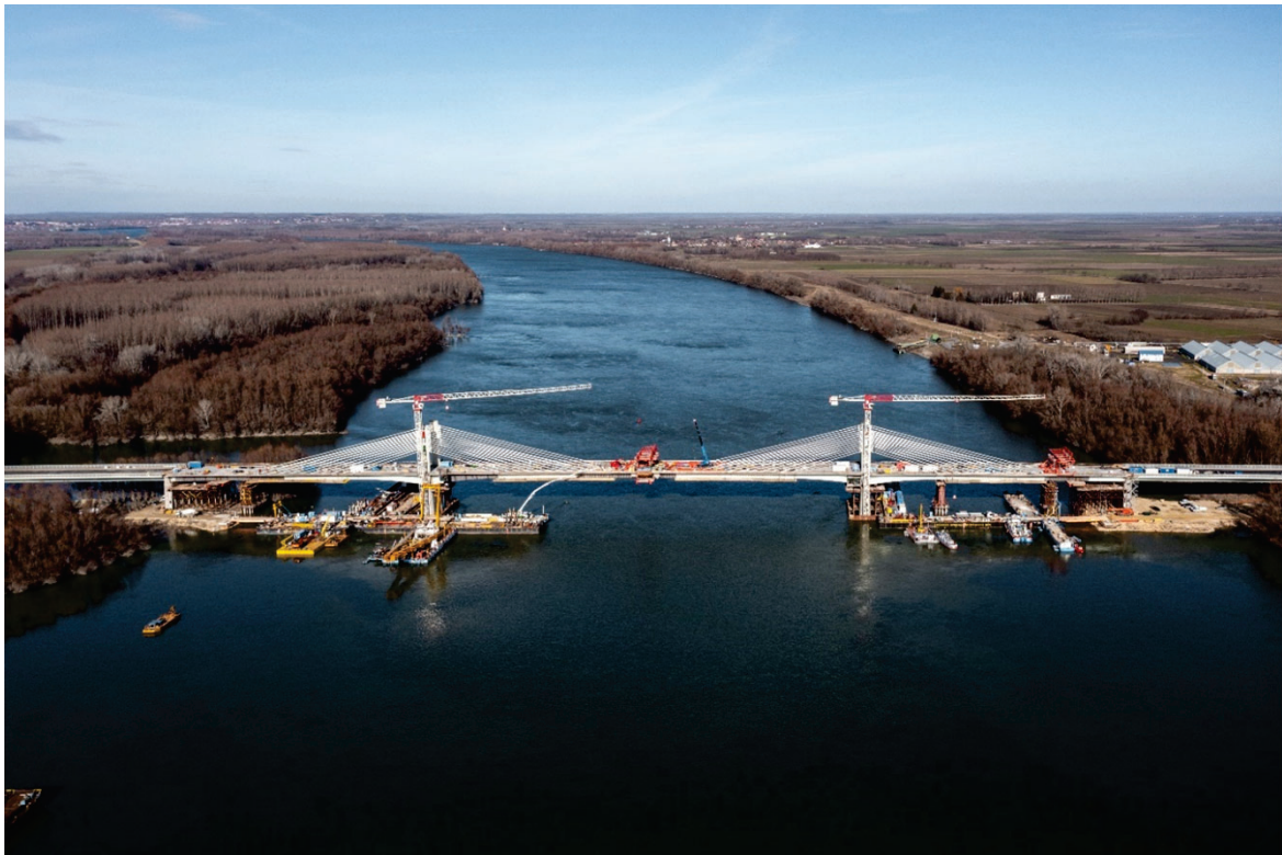
Figure 9: Cantilever construction of the river bridge (photo: Tamas Dernovics magyarepitok.hu)
