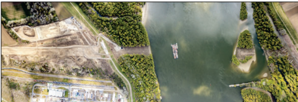
Figure 1: Aerial view of the worksite, foto: Mihaly Erdei magyarepitok.hu
