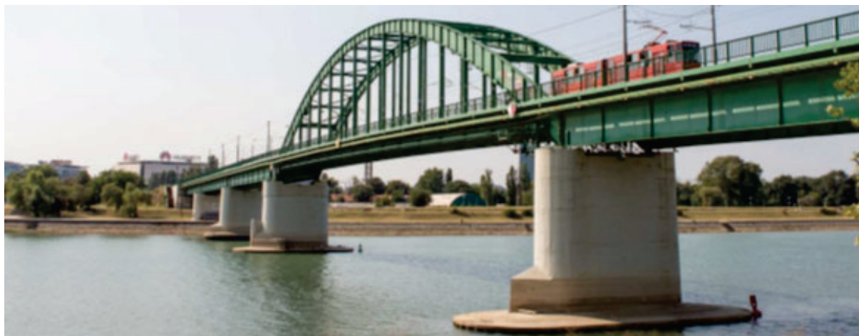
Figure 4: Old Sava Bridge at present
