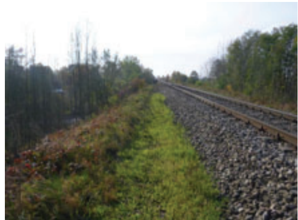
Figure 3: Schwillach dam at km 26,0, South-west view
