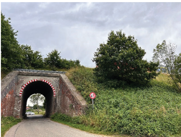
Figure 9: Existing Dorfstraße bridge
