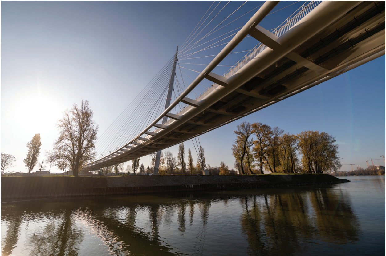
Figure 1: The Robinson Bridge is located at the confluence of the Danube and the Soroksári-Ráckevei Danube Branch (Source: Magyar Építőők)
