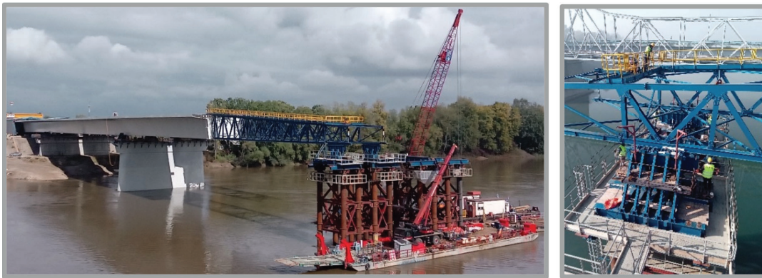
Figure 14: Temporary Pier D01
