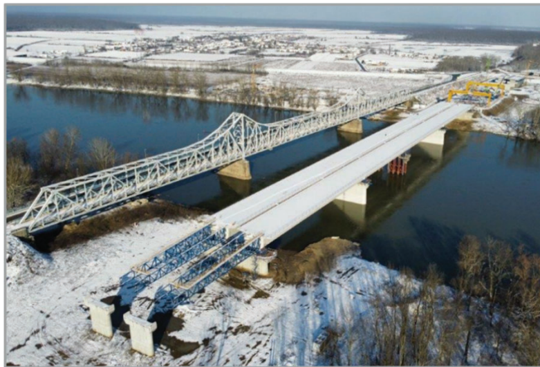
Figure 5: Launching of Bridge Structure
