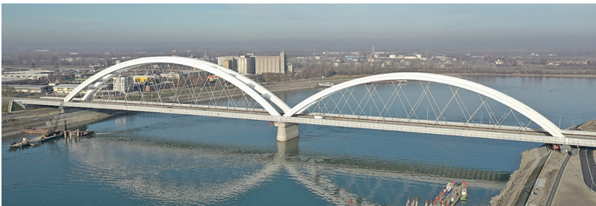
Figure 1a: Railway-Roadway Bridge across the Danube in Novi Sad – Downstream View [1]
