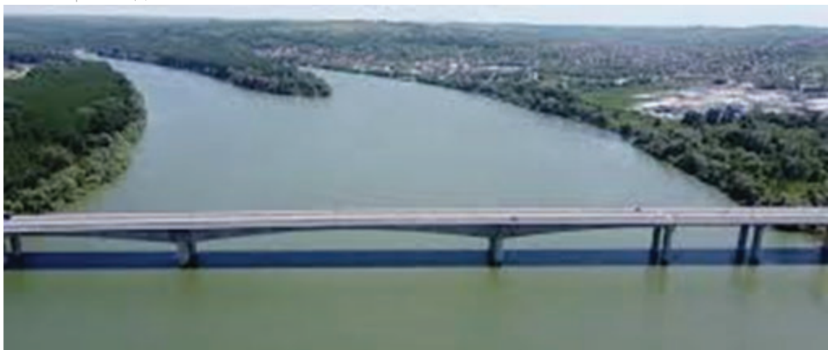
Figure 8: Highway Bridge across Sava River at Obrenovac – Side View, Cross Sections and Downstream Photo [8]
