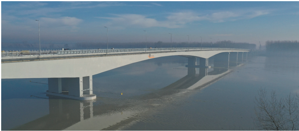
Figure 7b: Highway Bridge across Sava River at Šabac –Downstream Photo [7]
