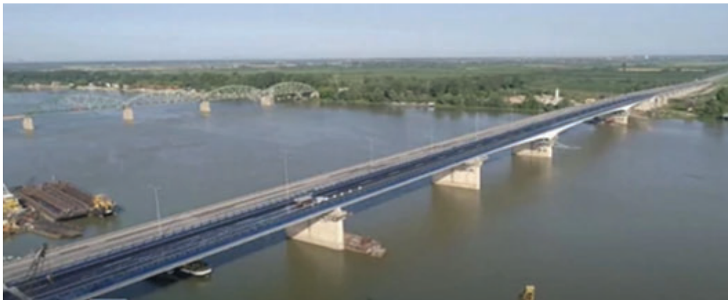
Figure 9: Highway Bridge across Sava River at Ostružnica – Side View, Cross Sections and Upstream Photo [9]
