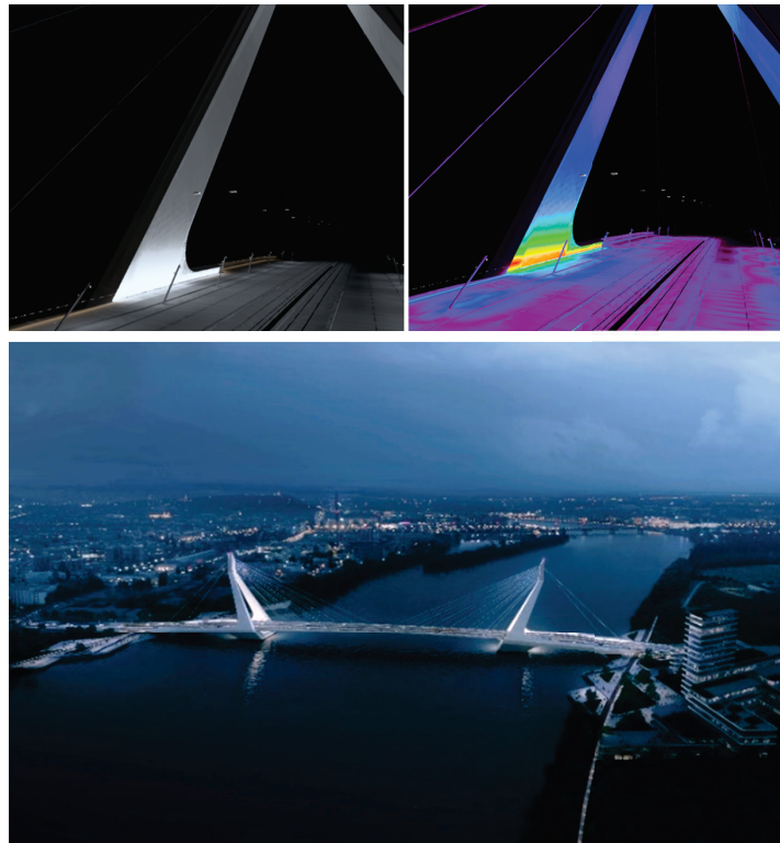
Figure 10: Render of pylon showing lighting intensity – © Buro Happold. Rendered night time image – © UNStudio / ZOA
