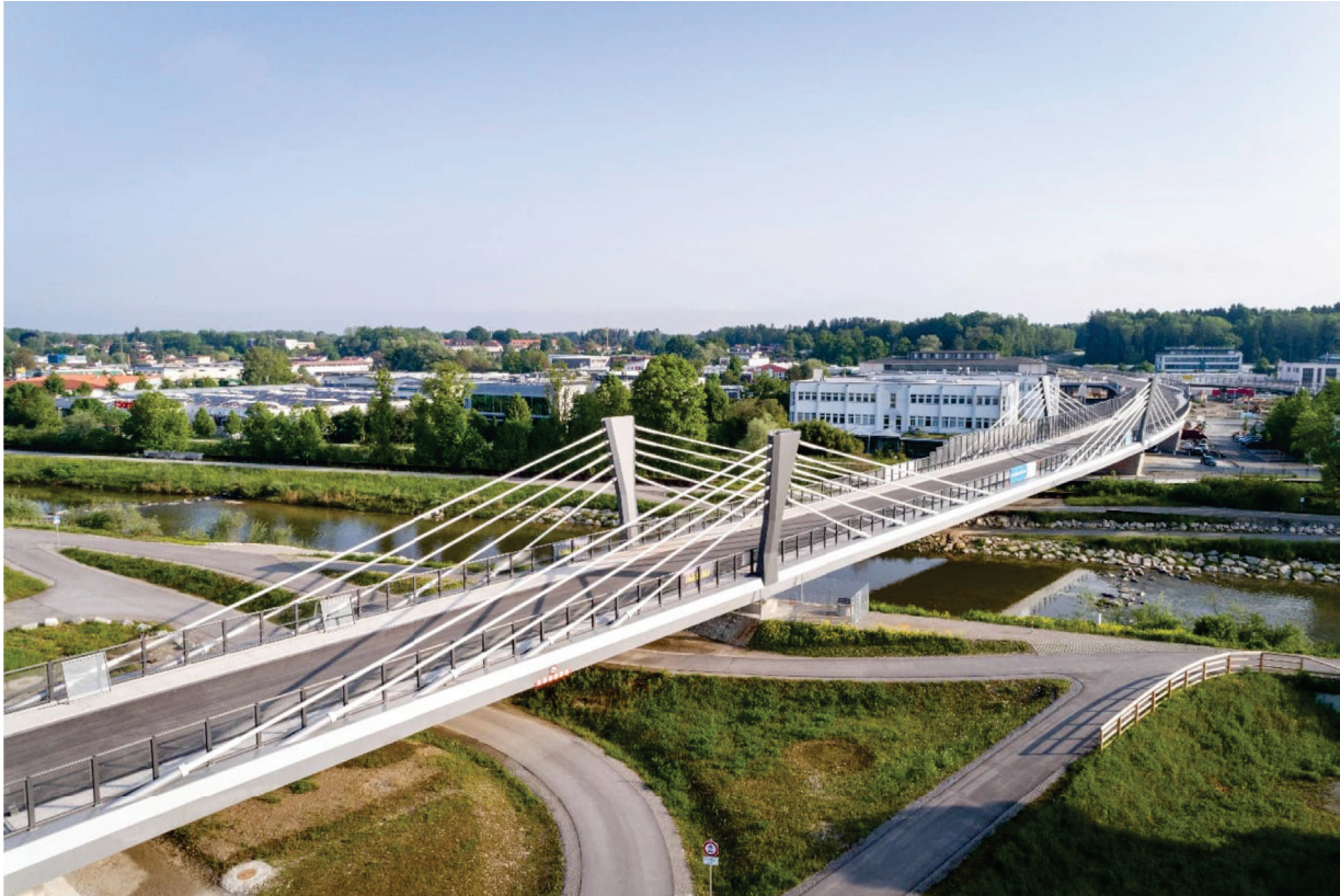
Figure 1: Oblique View of the Bridge Structure (©Ingenieurbüro Grassl GmbH, photography Stefan Kuhn)
