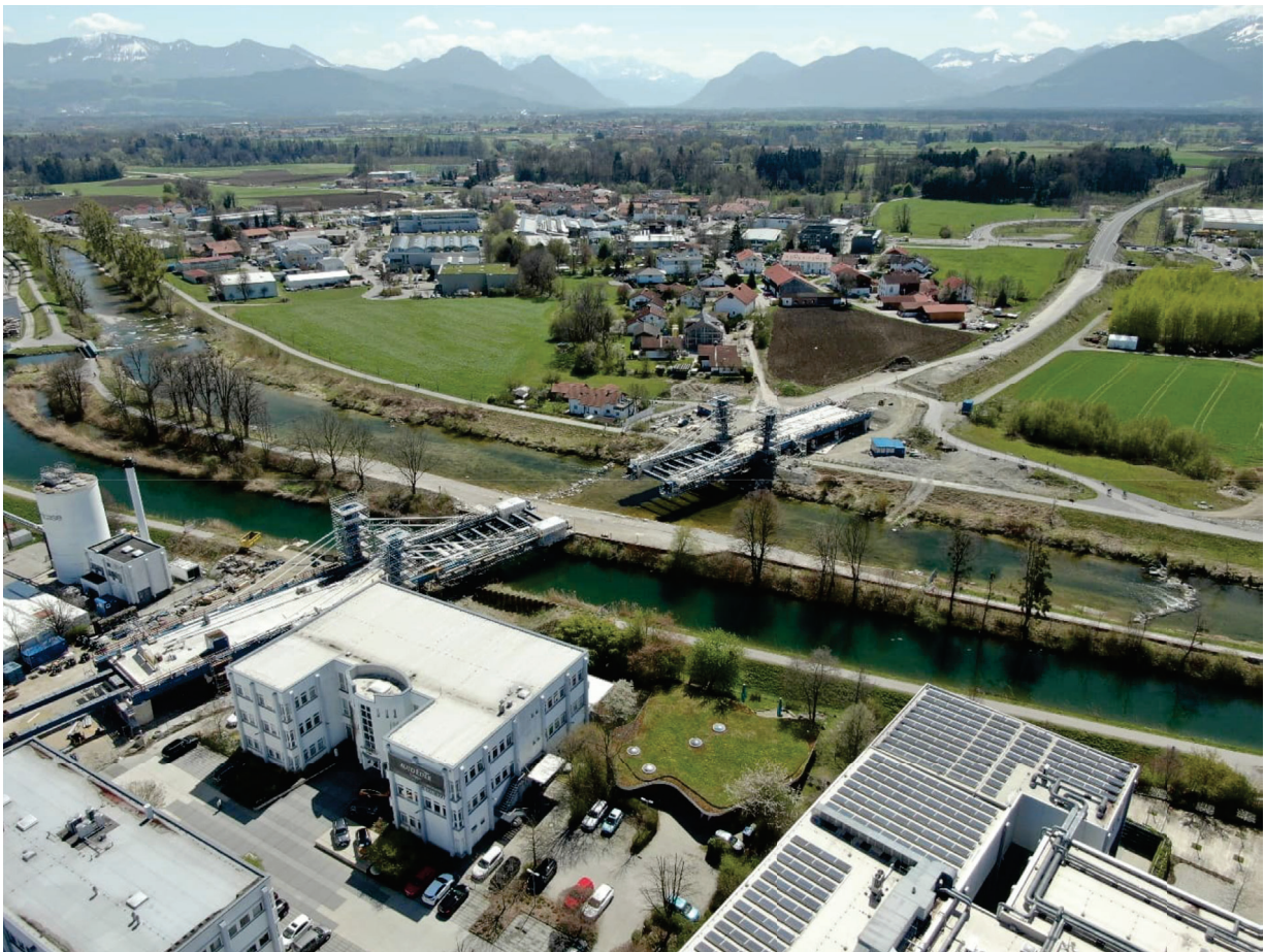
Figure 11: Free Cantilever Construction in Front of Mountain Scenery (©Ingenieurbüro Grassl GmbH)
