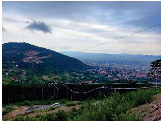
Figure 14: Towing of the main cables
