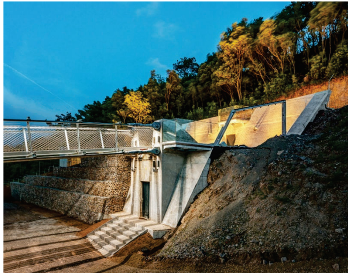
Figure 10: Photo of the almost ready abutment on Várhegy (by Attila Gulyas)
