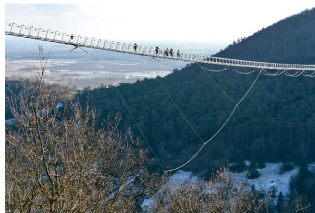
Figure 16: Lowering the wind cable system
