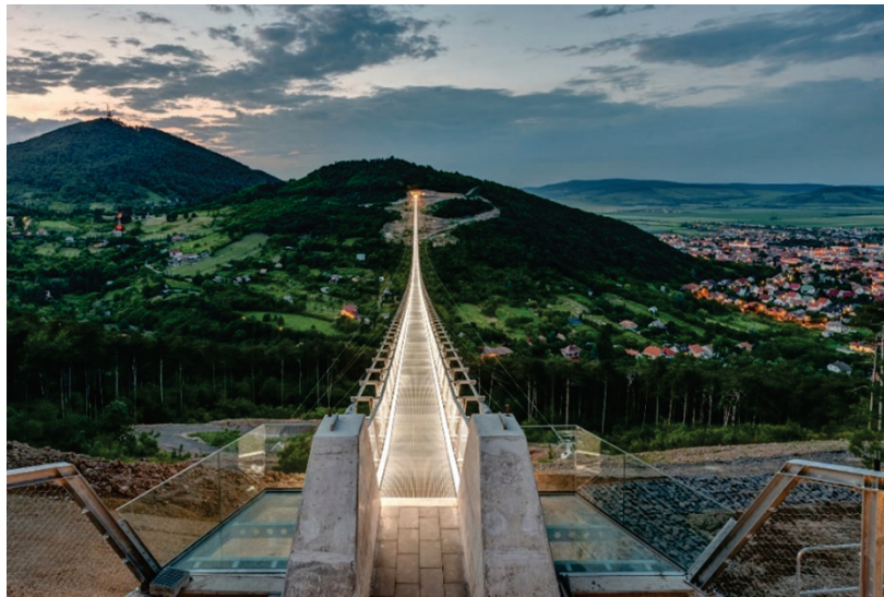
Figure 11: Top view of the illuminated bridge (by Attila Gulyas)
