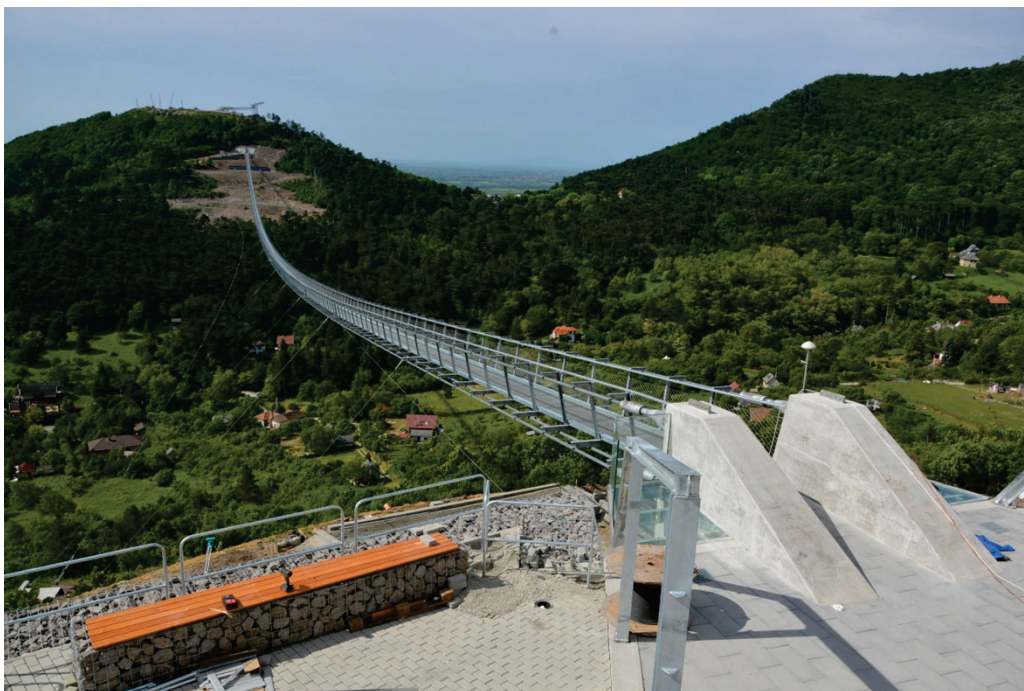
Figure 5: Global view of the almost ready bridge
