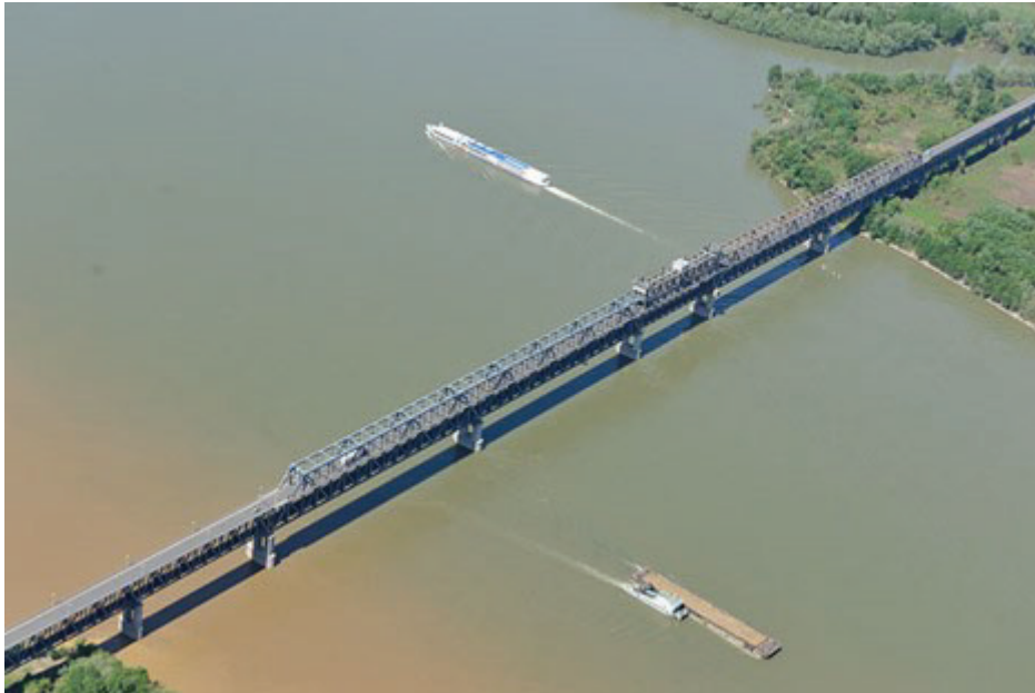
Figure 1: General overview of the bridge [2]
