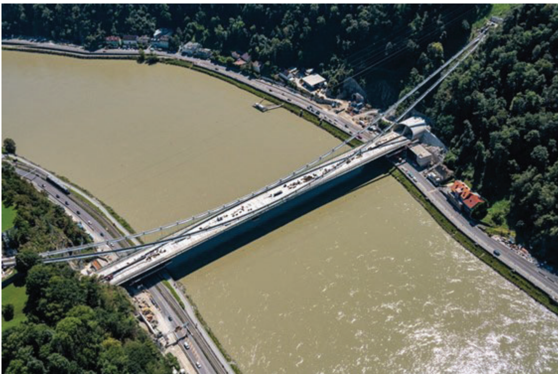
Figure 5: Bridge Deck / ASFINAG
