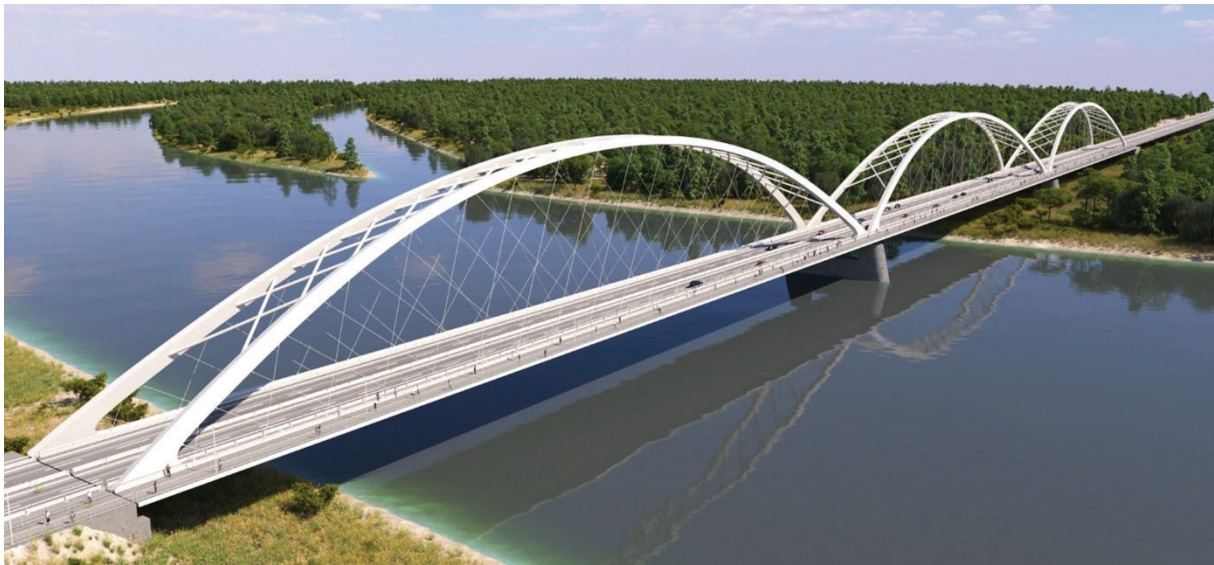
Figure 2: The bridge structure is series of three network arches
