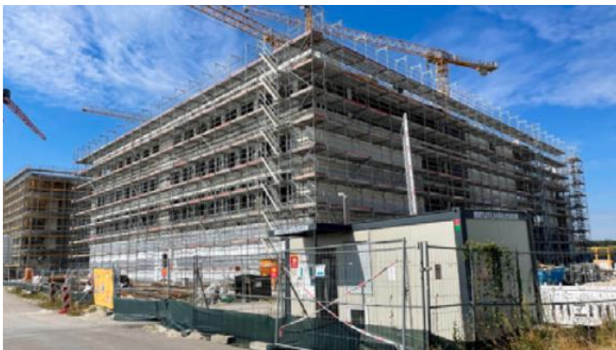
Figure 13: On-site environment of case study building
