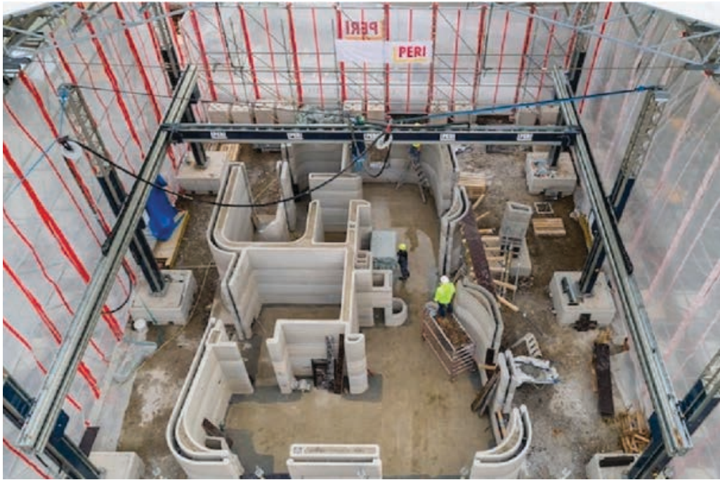
Figure 2.4: On-site printing with a gantry system (F. P. Bos et al., 2022)
