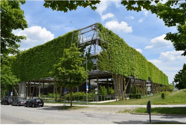
Figure 2 Ground-based growth on climbing aids (Swiss Re office building in Munich); (Source: Bundesverband GebäudeGrün)
