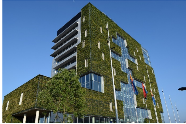
Figure 3 Wall-based modular system (living wall) (Municipality of Venlo, Netherlands); (Source: Bundesverband GebäudeGrün)
