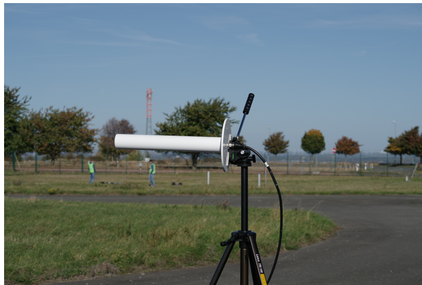
Figure 3. Jammer antenna installed on the ground.
