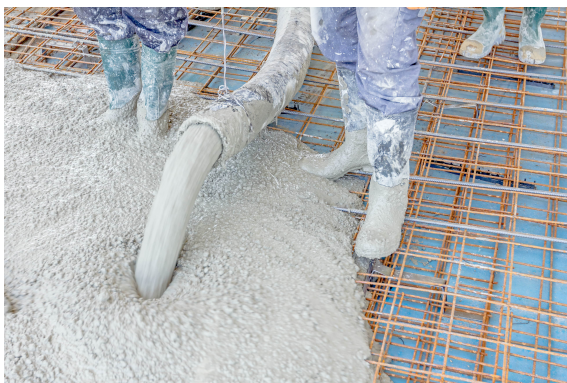
(c) Pumping of concrete
