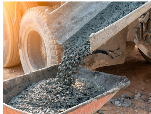
(b) Pouring of plastic concrete
