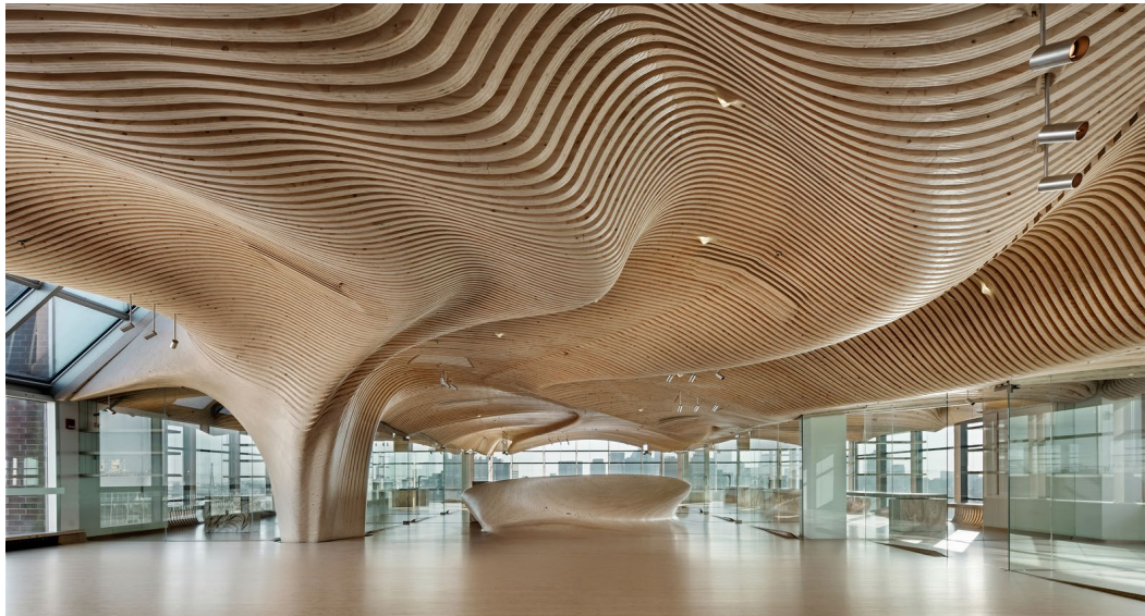
Figure 1: The interior renovation project was nested onto 1200 3.6m * 1.2 m plywood sheets and milled using a small 3-axis CNC router, dECOi Architects .
