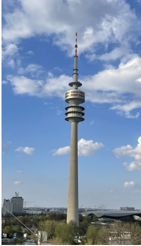
(a) Olympic tower
