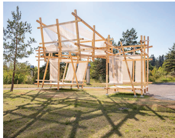
Figure 21: The reciprocal configuration allows high geometric complexity using only simple planar joints (©Ali Zigeli 2022).
