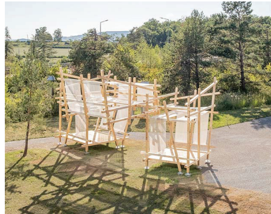
Figure 1: The Cantibox project leverages innovative approaches to structural design and robotic assembly to enable the development of a customized spatial timber structure (©Ali Zigeli 2022).
