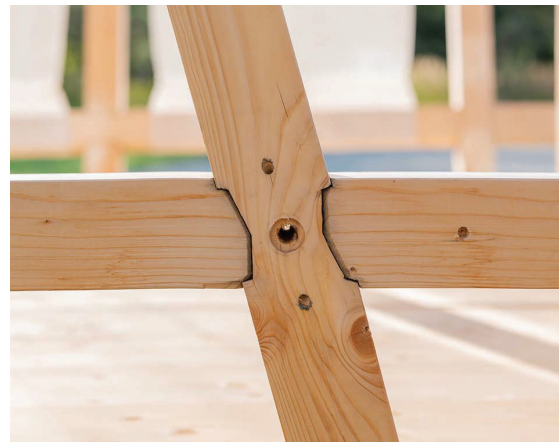
Figure 15: CNC machines foster the design of bespoke geometry for the connections. All the half-lap connections – prototypical and bespoke – are machined with a Hundegger Robot Drive automatic joinery machine (©GKR 2022).
