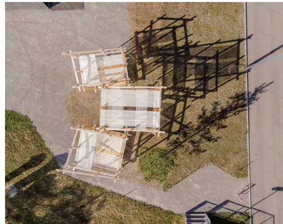
Figure 20: The CantiBox is partially covered with translucent fabric to provide shading (©Ali Zigeli 2022).
