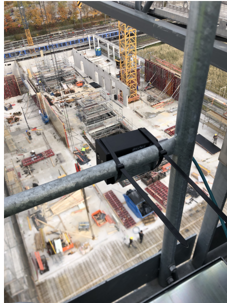
Figure 5.1: Scanner fixed to crane on real construction site
