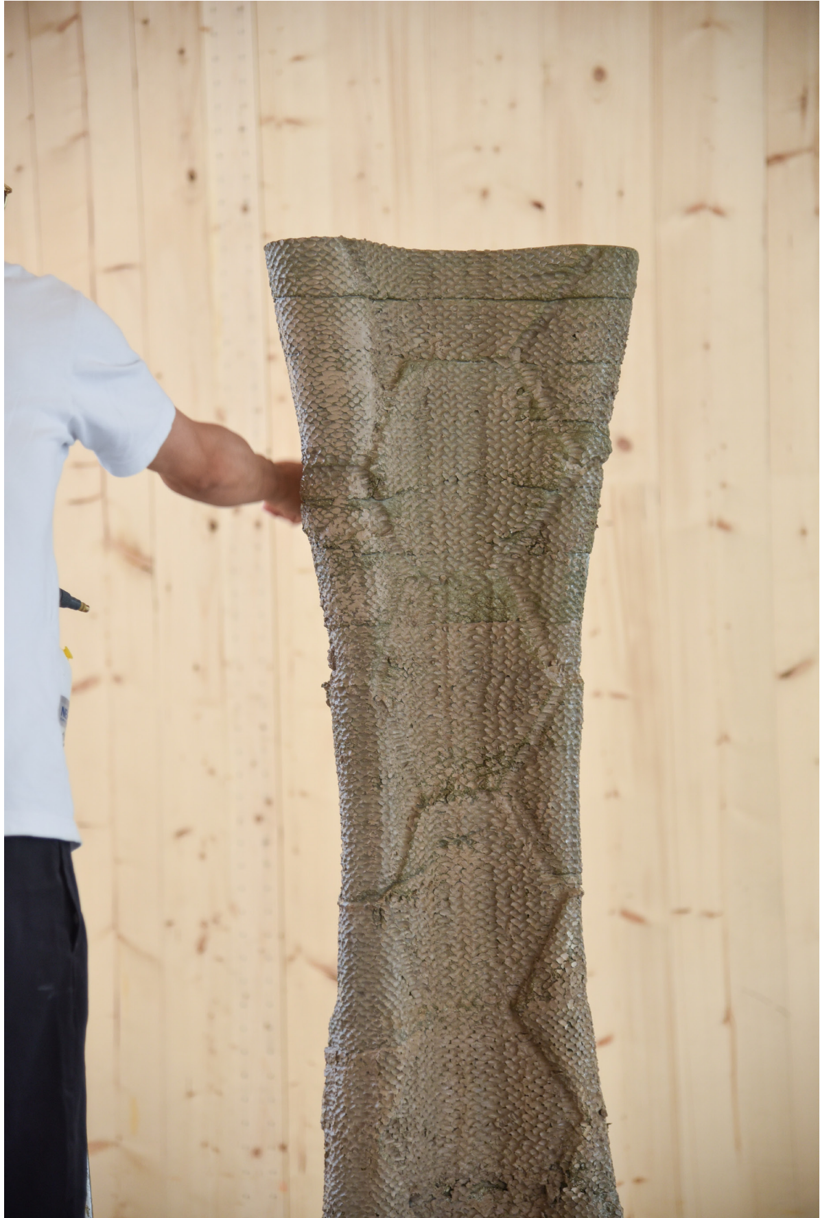
Figure 43: Finished concrete column. The undulation of print path left a texture on the concrete surface. The joints also leave marks on the concrete. Picture credit: Gido Dielemans
