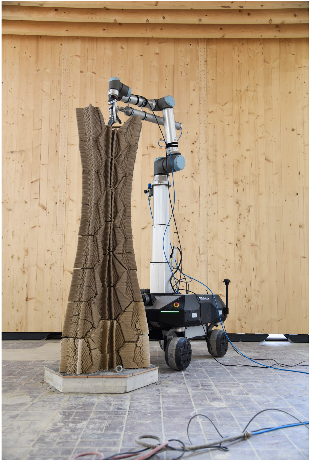
Figure 39: Clay formwork of the column being printed. Photo credit: Gido Dielemans
