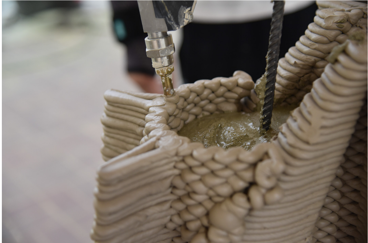
Figure 42: Clay formwork being printed. Picture credit: Gido Dielemans
