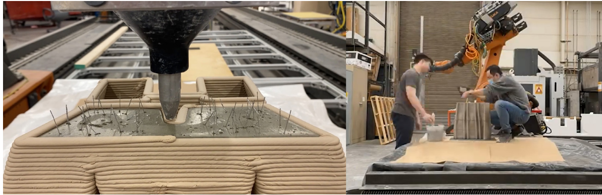
Figure 3: Clay formwork being printed on top of previous cast (left). (“Print-Cast-Print - YouTube” n.d.) Concrete being casted in 3d printed clay formwork (right). (“3D PRINTED CLAY FORMWORK FOR CONCRETE CASTING - YouTube” n.d.)
