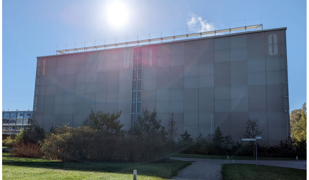
Leibniz Supercomputing Centre (LRZ)
