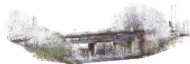
Figure 6: Original point cloud of bridge
