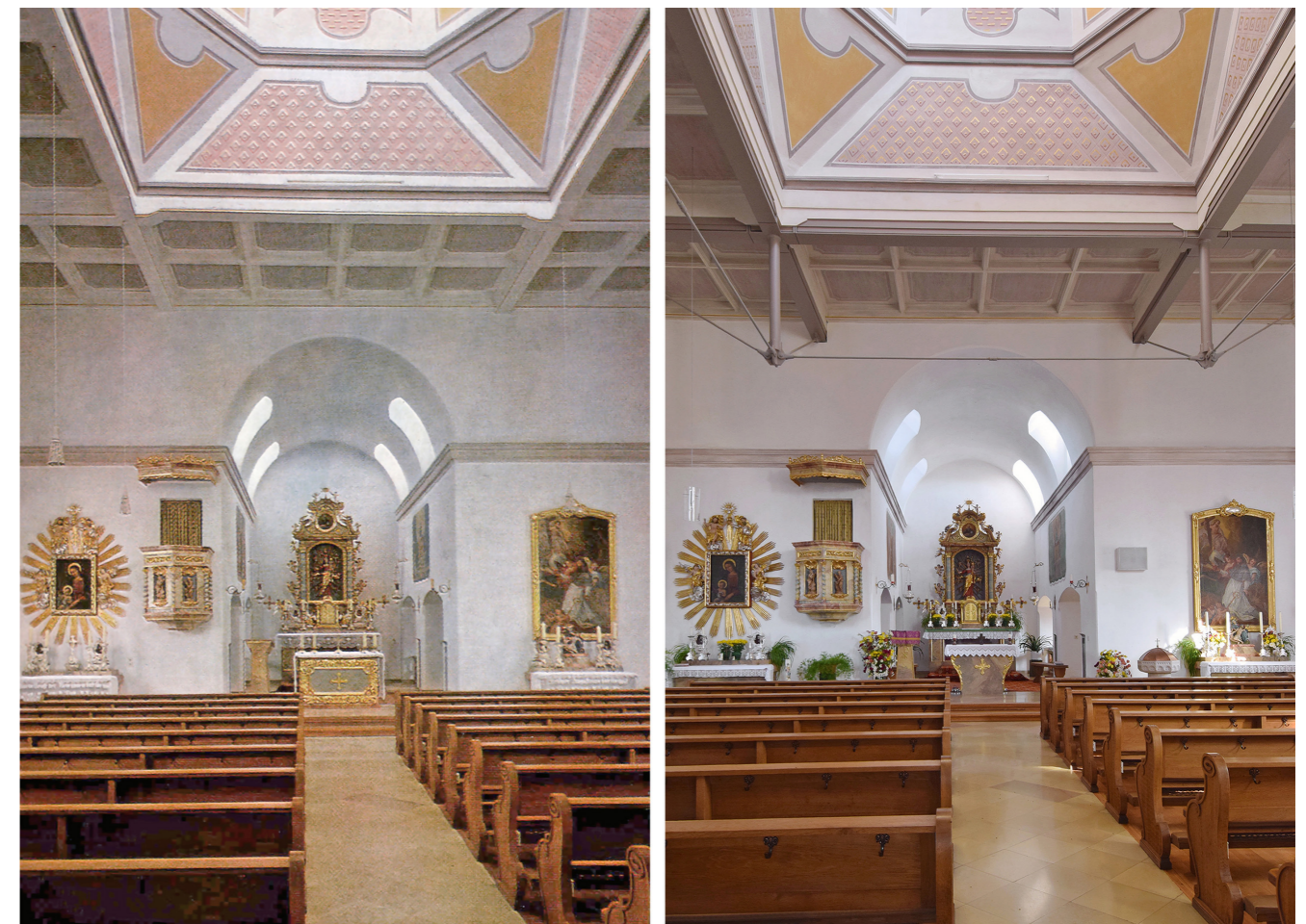
Fig. 10: Interior view in comparison before and after repair (Peter Kifinger)
