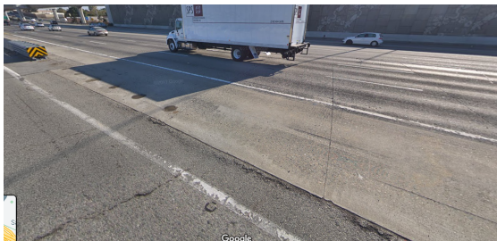
Figure 4.1: Center divider, marked with badly painted lane markings, of the crash [38].
