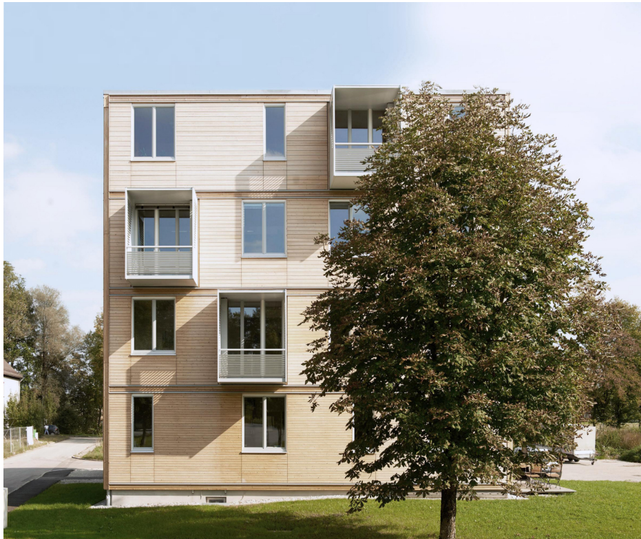
Figure 14: four-storey residential building developed in a research project together with the Technical University of Munich, the Rosenheim University of Applied Sciences and the ift in Bad Aibling. The building's entire supporting structure is made of wood and is self-stiffening without any concrete parts. Ceilings and walls, lift shaft and loggias are also made of wood. [62]
