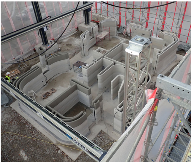
FIGURE 12 Germany's first 3D-printed house in Beckum, Westphalia, under construction. The tests for material approvals (ZiE) and the construction project-related type approval (vBG) were carried out at the Technical University of Munich. (pic: D. Weger)
