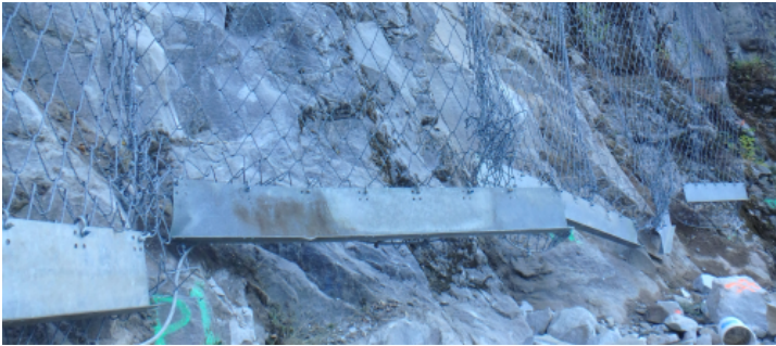
(a) Additional weight at the bottom of the protection net to ensure a more controlled structural deformation.
