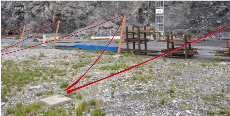
Figure 3.5: Depiction of the application of truss finite elements in the construction of the flexible protection structure. The columns highlighted in orange will be modeled with trusses. Entities highlighted in red will be modeled with cable elements, described in subsection 3.2.7.2. Photograph taken in Walenstadt, Switzerland.
