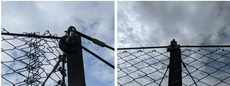
(a) Edge installation.
