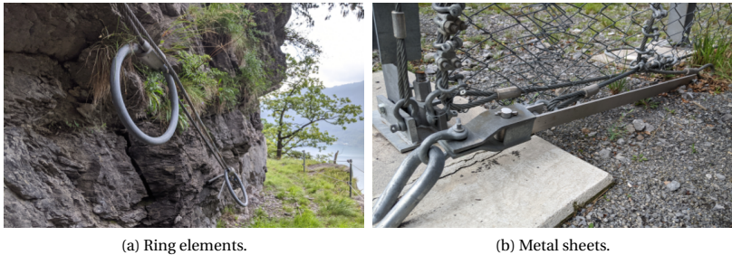
Figure 2.4: Photographs of the energy dissipation elements, taken in Walenstadt, Switzerland.
