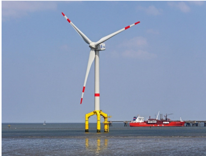
Figure 2.2: An offshore wind turbine [44]
