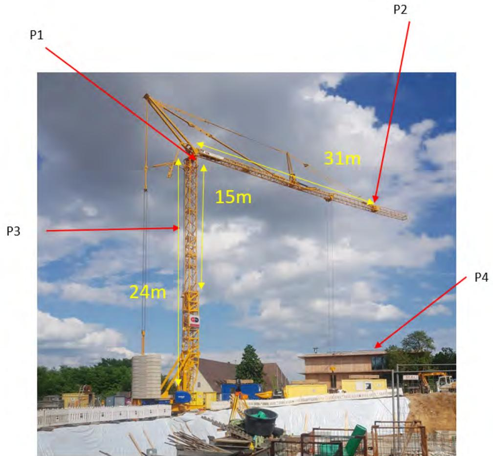
Figure 5.10: Positions of crane cameras
