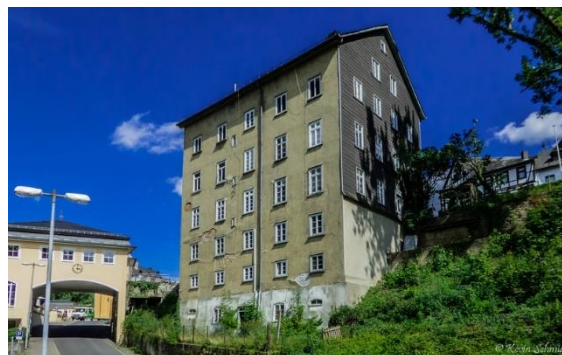
Fig 2.4. Hainallee 1 Weilburg, the highest pisé house in the world
