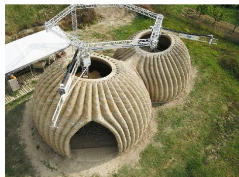
Fig 2.13. 3D-printing process by Wasp 3D
