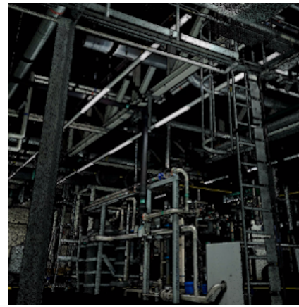
Figure 9: Real laser scan point cloud of the facility, with actual RGB values
