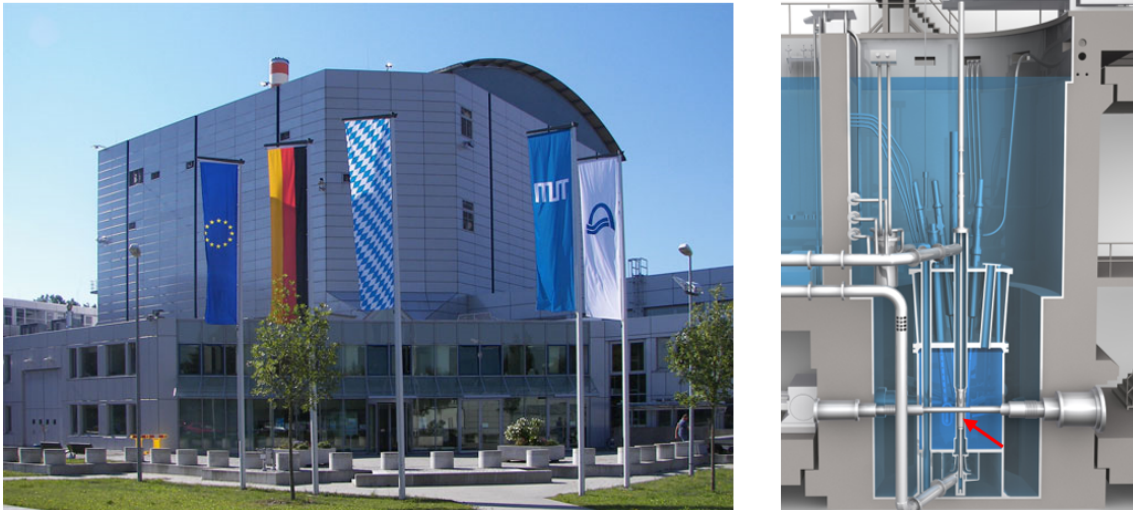
FIGURE 1.1: Left: overview of FRM II. Right: section of the reactor pool. The fuel element in the central channel is indicated by the red arrow. [4]
