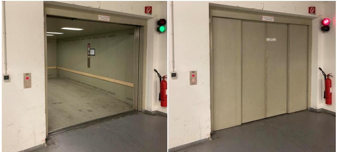
Figure 4.6: Elevator (Own photograph)
