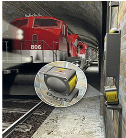
Figure 2.4: Train detection in tunnel with the help of radar sensor (Banner Engineering Corp., 2017)
