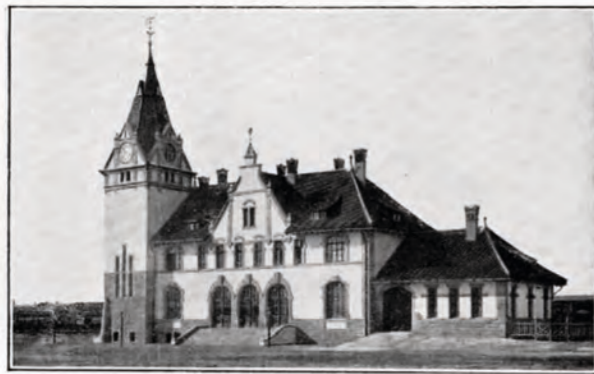
Figs. 2a & 2b, top: A depiction of the original structure in Führer durch Tsingtau und Umgebung by Behme and Krieger (Wolfenbüttel: 1904); Bottom: Reconstructed Qingdao railway station in 2018 (Falser 2018).
