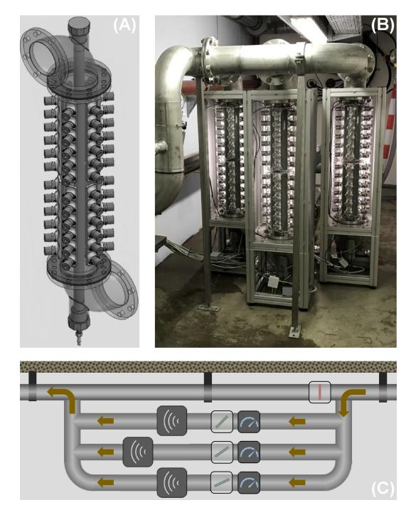
**Figure 7.1:** 3-D schematic of the employed double-tube reactor (A), photograph of the whole reactor setup (B), and top view assembly plan of the reactor installation (C). The closed value in the main waste activated sludge (WAS) pipe is indicated by a red bar, while the partially opened values in the inlet pipes to the ultrasound reactors are indicated by green bars. WAS flow is indicated by brown arrows.
