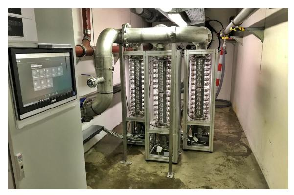
**Figure 10.1:** Photograph of the full-scale US reactor system depicting individual reactors, pipes, and the control cabinet at the Starnberg wastewater treatment plant.
