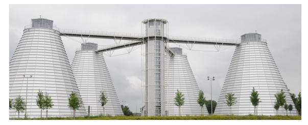
**Figure 1.1:** Anaerobic digesters at the Gut Großlappen WWTP in Munich, Germany (photographed by Philipp Weigell<sup>1</sup>).
