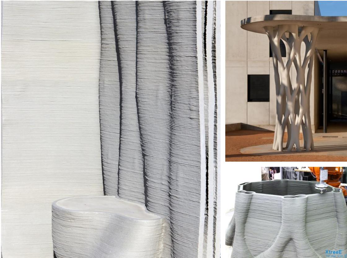
Figure 9: Sinusoidal wall with internal 3D sinusoidal shell printed by XTreeE (left) and post for a school in Aix en Provence printed with temporary supports and as lost formwork (left) (XtreeE, 2016)
