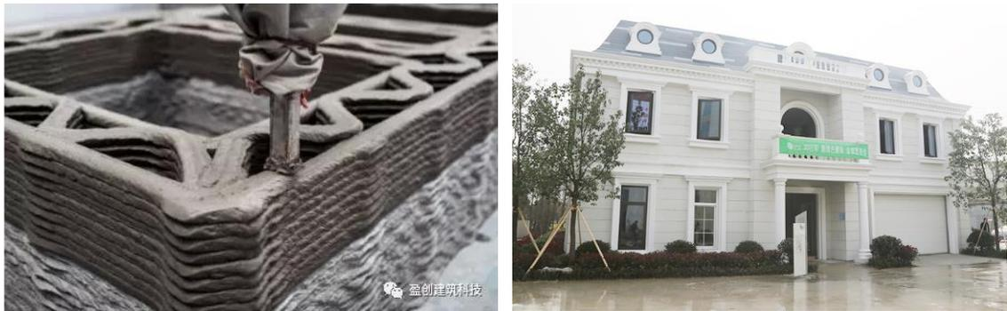
Figure 7: Offsite extrusion-based printing of concrete elements with internal zigzag structure (left) and 3D printed villa on the WinSun company property (right) (WinSun3D, 2020)
