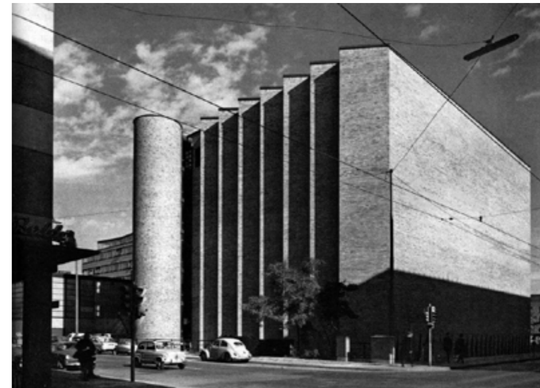
The High Voltage Haus of the faculty of Electrical Engineering
