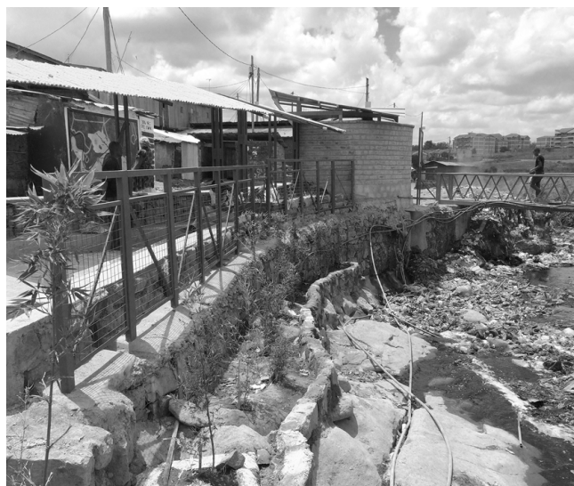
Figure 6. River remediation and flood protection project developed at Andolo with residents using flood model outputs (photograph: Jack Campbell Clause, KDI)
