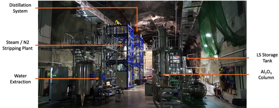
**Figure 4.5:** Photo of the pilot plants as they were installed in the LS Hall in Daya Bay in 2016/17. In the foreground, the water extraction system (left) and the filtration facility (right) can be seen. Behind them (on the left) are the stripping and distillation units in their blue assembly frames.
