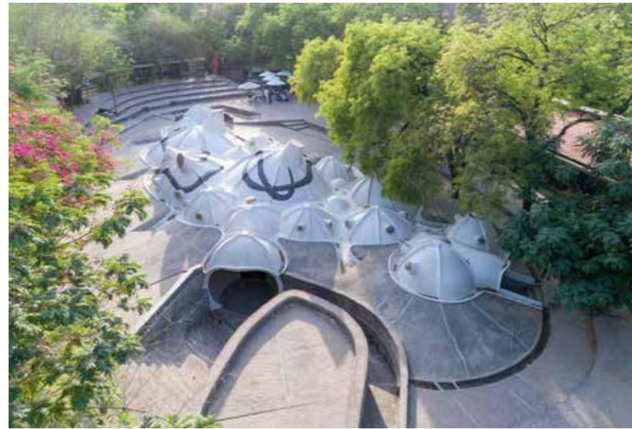
Detail view of the roof landscape of the "Amdavad Ni Gufa" art space, Ahmedabad, 1994. © Ivan Baan 2018
